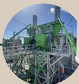
New batching plant Hal Far
